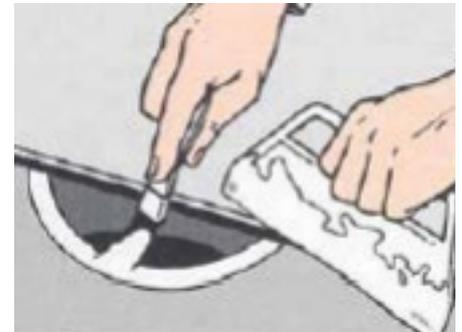
Heat the floor covering gently and fit it into the floor drain. Fit the clamping ring and double check the adhesion for water tightness. The edge of the installed floor covering should then be sealed.
