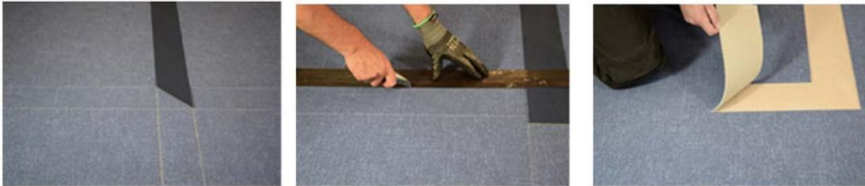
Apply a fresh layer of acrylic adhesive. Lay the Artline border into the adhesive after the appropriate waiting time specified by the adhesive manufacturer and using a rubbing board press the border firmly into the adhesive (see below).
