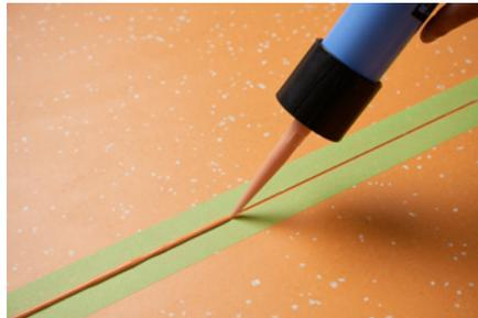
5. Immediately after application, the cold weld is pressed into the joint with the nora<sup>®</sup> smoothing spatula by running this evenly over the joint. Thereby, the surplus cold weld is pressed to the left and right of the joint. Hold the spatula in a position as flat as possible to avoid the development of hollow joints.
