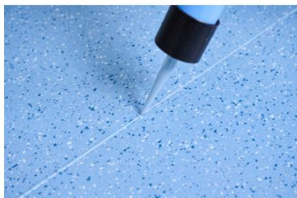
5. Immediately after application the cold weld is pressed into the joint with the nora<sup>®</sup> smoothing spatula by running this evenly over the joint. Thereby, the surplus cold weld is pressed to the left and right of the joint. You have to make sure that the cold weld pressed to the sides is entirely separated from the compound in the joints. Hold the spatula in a position as flat as possible to avoid the development of hollow joints.
