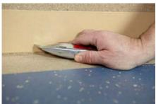
Cut cushioned-edge profile to size – use the nora<sup>®</sup> profile cutter to cut the outer and inner edges to mitre – and fix the profile.
