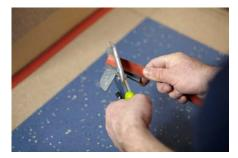
Place nora<sup>®</sup> profix 90 max. 2 mm from the floor covering edge and rub thoroughly into place.
