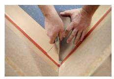
**8.** Cut the floor covering strips required for the skirting formation to size (width 19 cm).
