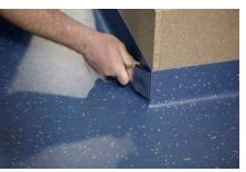
12. The seams to the previously installed floor covering have to be joint-sealed. This can be done either with nora® hot welding rod 24 hours after installation or with nora® 1-component cold weld directly after the installation (see processing recommendation "Joint sealing").
