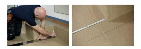
2. Position noraplan<sup>®</sup> and cut the seams. Apply adhesive exactly up to the marking and install the floor covering after airing.
