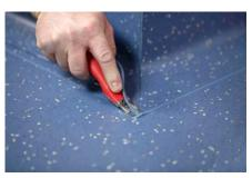
13. The inside and outside corners as well as the butt joints have to be jointsealed with nora® 1-component cold weld. This can be done directly after the installation and the application of nora® liquid wax (see processing recommendation "Joint sealing").
