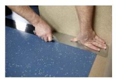
Fix nora<sup>®</sup> profix 90 to the wall and rub thoroughly into place. Cut off approx. 2 cm of the protective paper and remove it.
